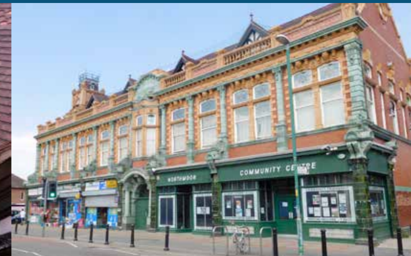
Restored to its former glory!
