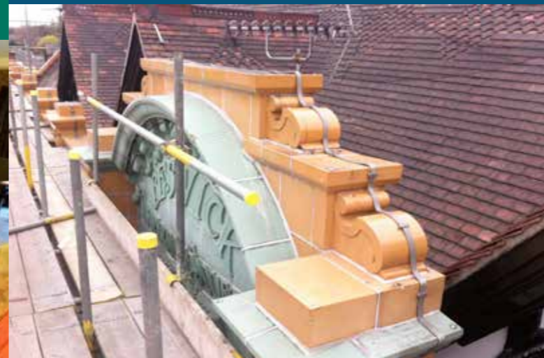
The Beswick Co-operative building mid-repairs
